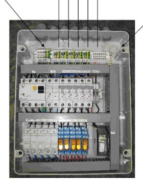
The merging box should not be used in case, that for connection of the outputs from the automat to heavy current wiring will be used stranded wires (eg. PNLY)
